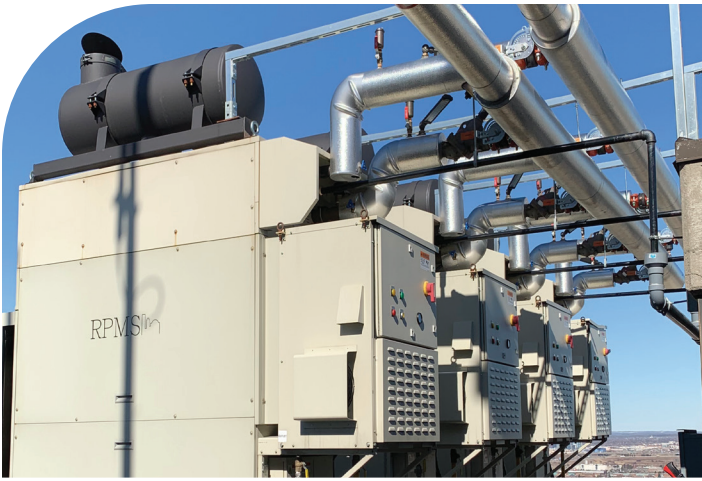
Four dual-mode ICHP Capstone C65 microturbines generate more than 1.9 million kWh per year, or about 60% of the building's baseload.
